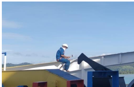
Gambar 4. 7 Chiping di Bowvisor Haluan tanpa Safety Harness dan Safety Googles
