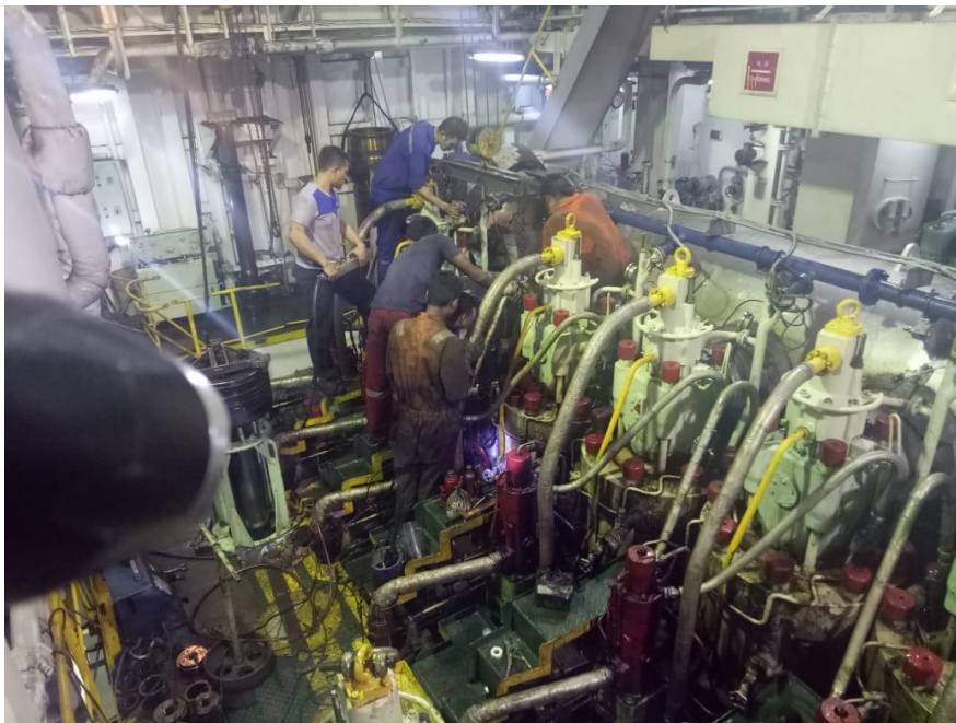
Lampiran 6. Overhaul Main engine
