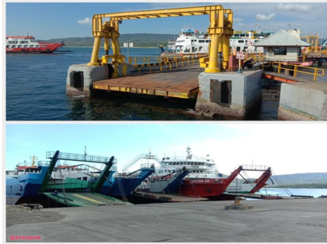
Gambar 4.19 Dermaga Ponton, Dermaga Moveable Bridge (MB) dan Dermaga Pelengsaan/LCM ( Landing Craft Mesin )
