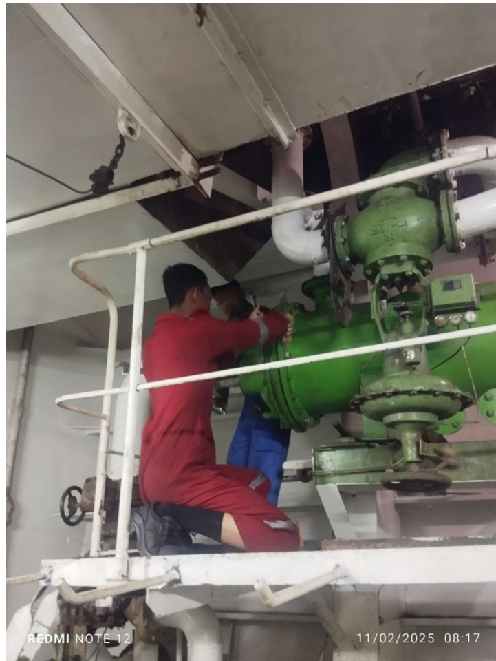
Lampiran 8 proses membuka cover fresh watre cooler
