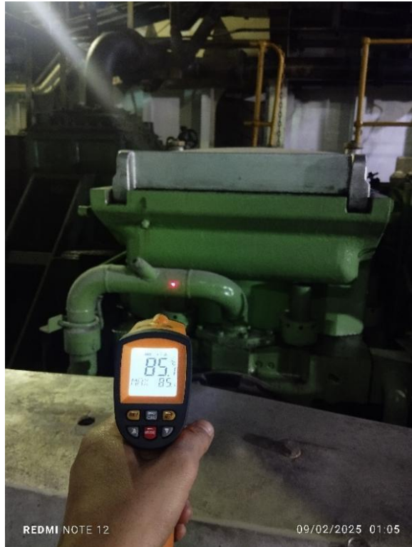
Lampiran 4 chek Temperatur pipa Fw outlet silinder no 8 sebelum perawatan
