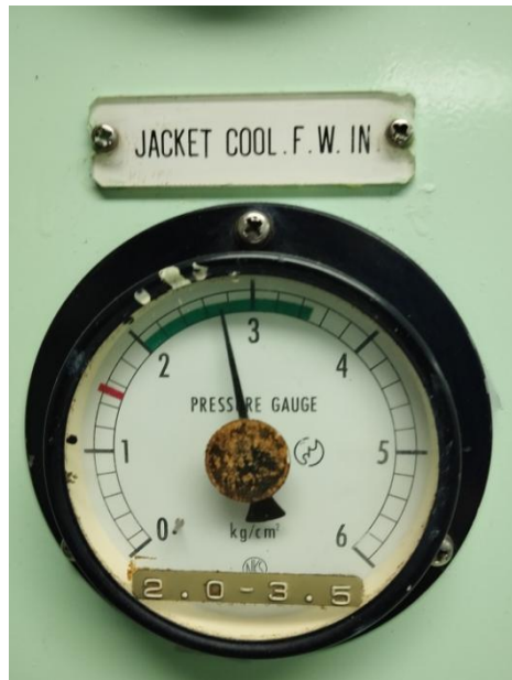
Gambar 4. 8 tekanan pompa fresh water normal
