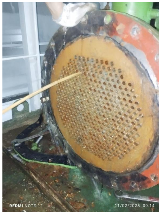
Lampiran 5 sogok cooler fresh water sebelum perawatan
