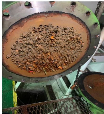
Gambar 4. 6 Fresh water cooler sebelum perawatan
