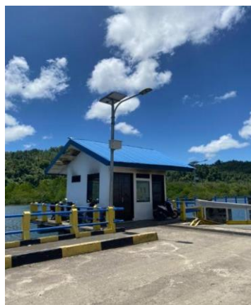
Gambar 4.13. Ruang Operator Movable Bridge
