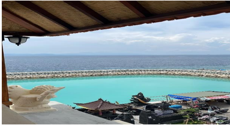
Gambar 4.12 Breakwater Pelabuhan Sampalan
