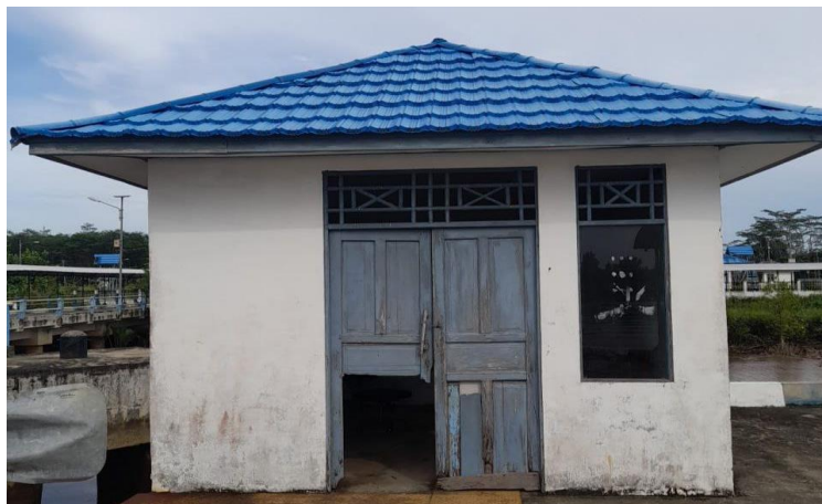
Gambar 4.9 Ruang Operator Movable Bridge
