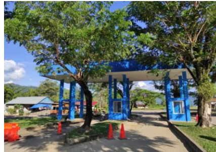
Gambar 4. 14 Toll Gate Kendaraan
