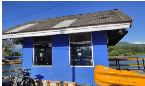
Gambar 4. 16 Rumah Moveable Bridge
