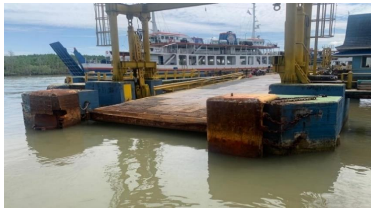
Gambar 4.17 Dermaga Movable Bridge Pelabuhan Kariangau
