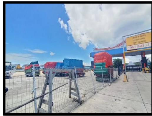
Gambar 4.43 Toll Gate eksisting
