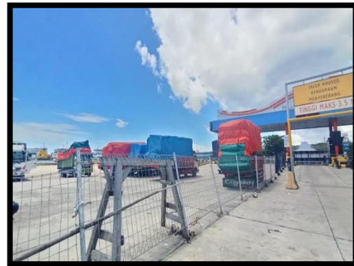
Gambar 4.43 Toll Gate eksisting
