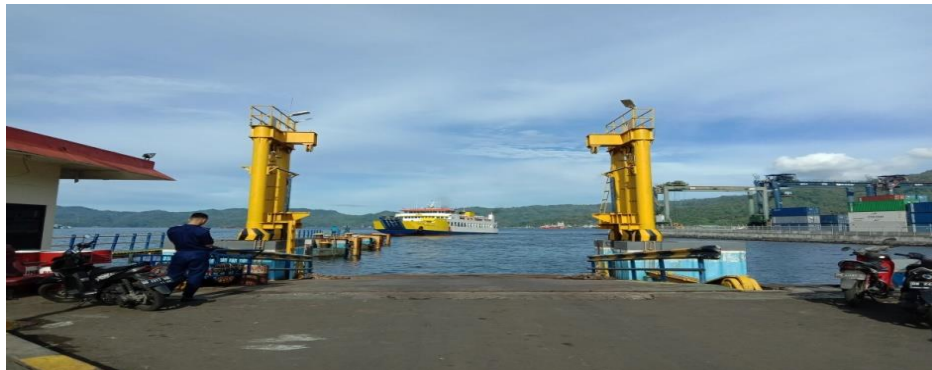
Gambar 4.11 Dermaga Moveable Bridge di Pelabuhan ferry ASDP Bitung
