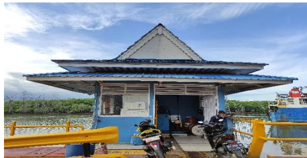
Gambar 4. 33 Rumah Operator Movable Bridge
