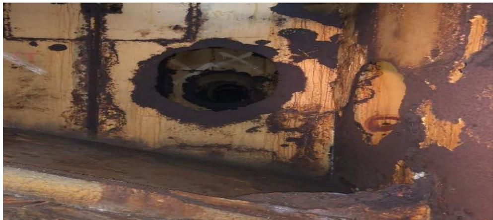
Gambar 4.32 Korosi di Sisi Bagian Dalam Kapal KMP Uma Kalada
