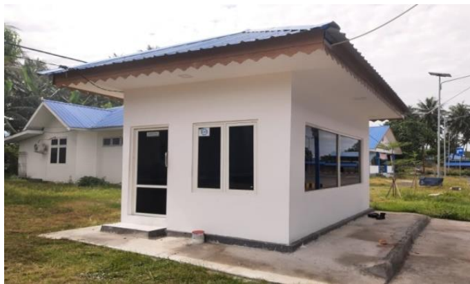
Gambar 4. 20 Rumah Moveable Bridge
