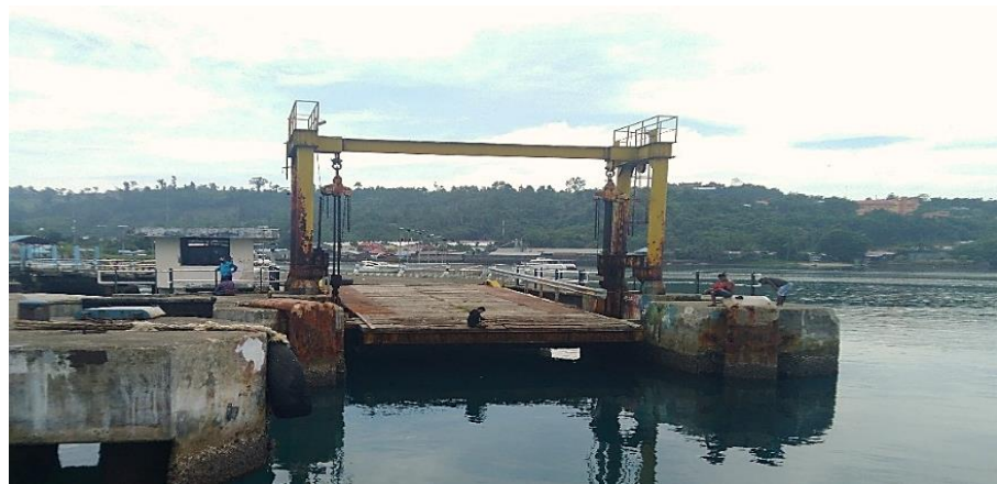
Gambar 4.12. Movable Bridge Pelabuhan Marampa
