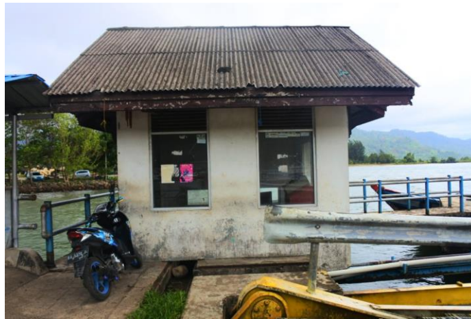
Gambar 4.7 Rumah Movable Bridge
