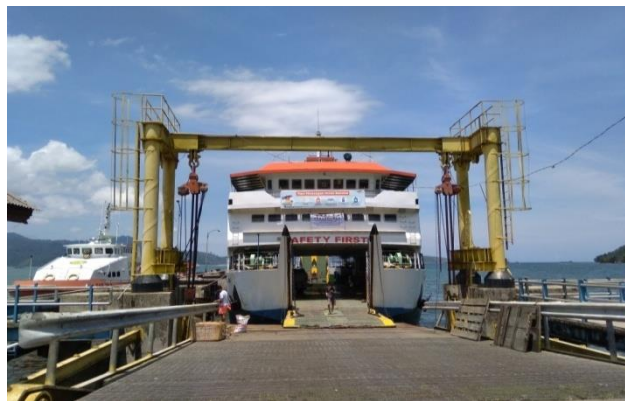
Gambar 4.4 Dermaga ( Moveable Bridge )
