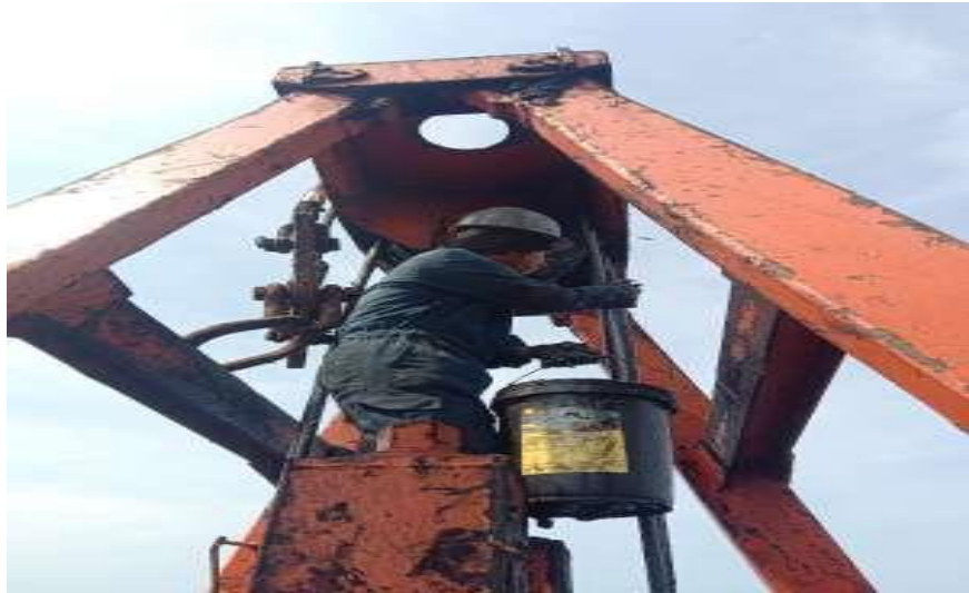
Gambar 4. 1 Greasing wire grab
