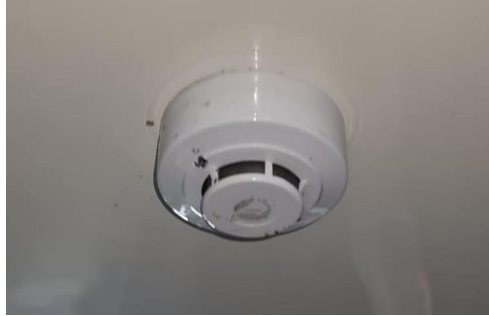
Gambar 4. 11 FFA Smoke Detector KMP. Barau
