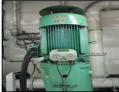
Gambar 2.3 LT Cooler Pump
