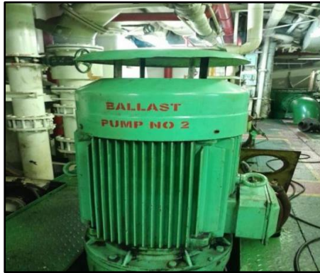
Gambar 2.1 Pompa Ballast
