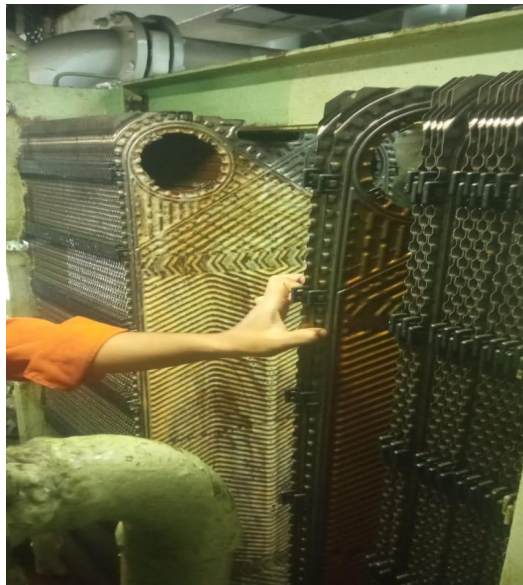
Gambar 4.3 Plat-plat pendingin Fresh Water Cooler
