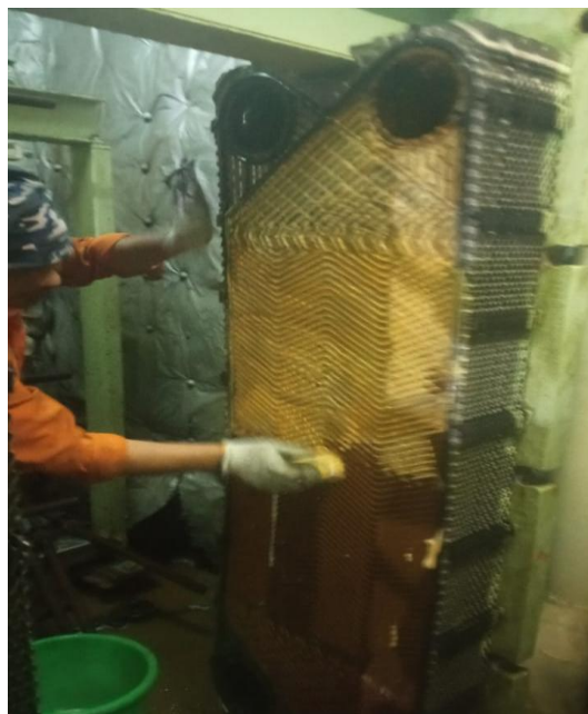
Gambar 4.4 Fresh Water Cooler saat dilakukan perawatan
