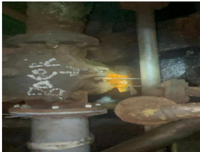
Gambar 4.7 Kebocoran Pipa
