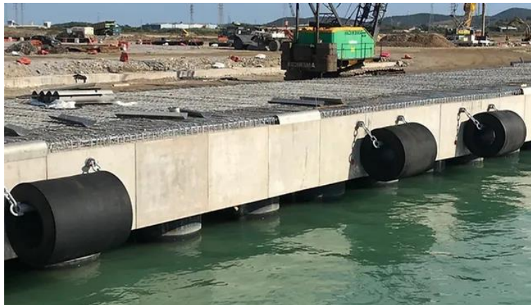
Gambar 2. 9 Fender Silinder FR2
