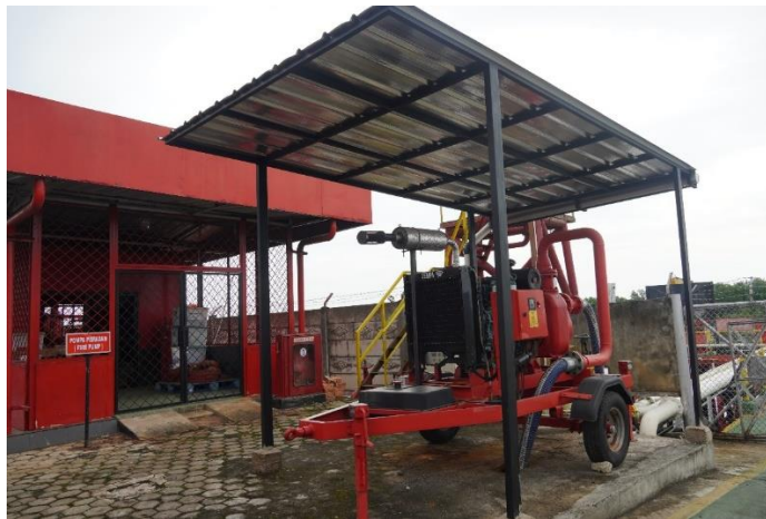
Gambar 4. 15 Pompa Intake
