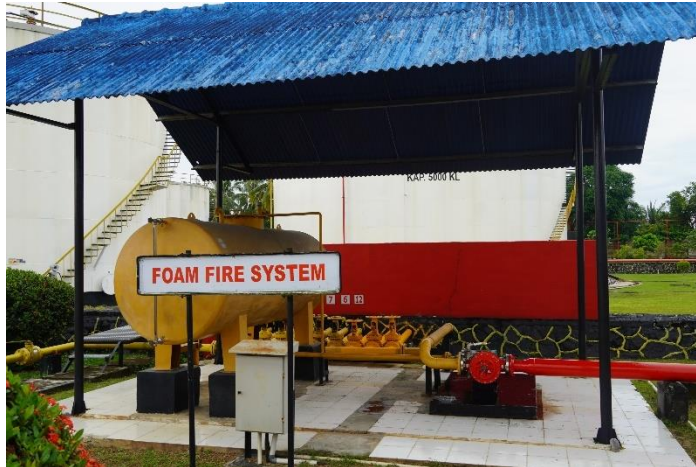
Gambar 4. 26 Foam Fire System
